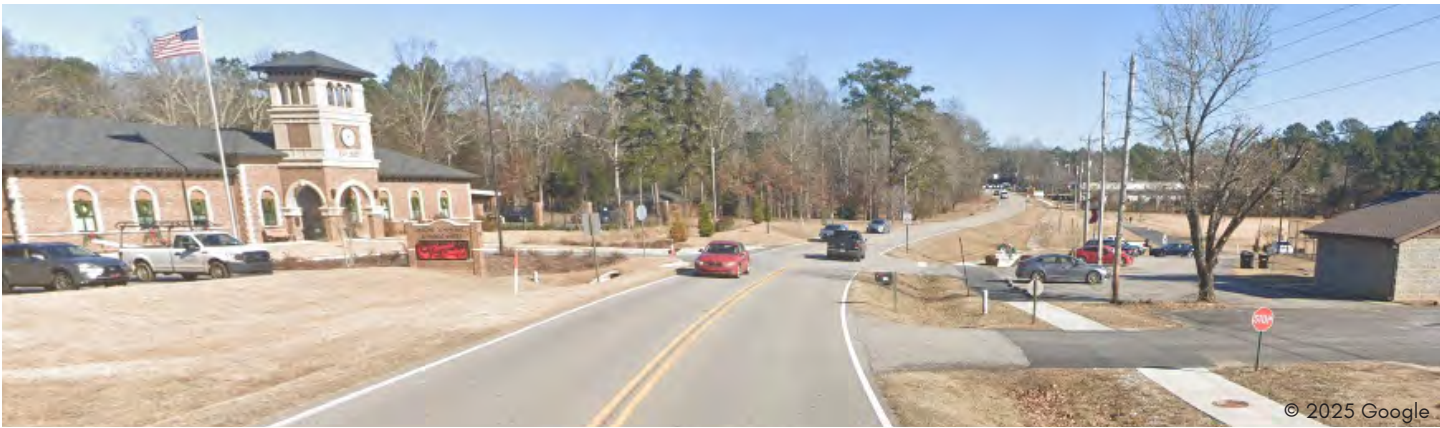
Current conditions on Senoia Road, facing east in front of Town Hall
